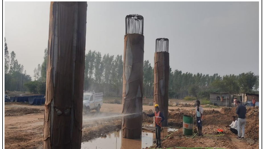
Pier Shaft RHS MJB 352+281 Curing work in Progress
