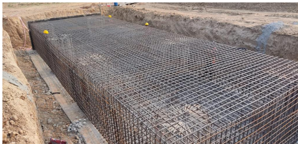
Reinforcement binding WIP of Pile Cap at MJB 352+281
