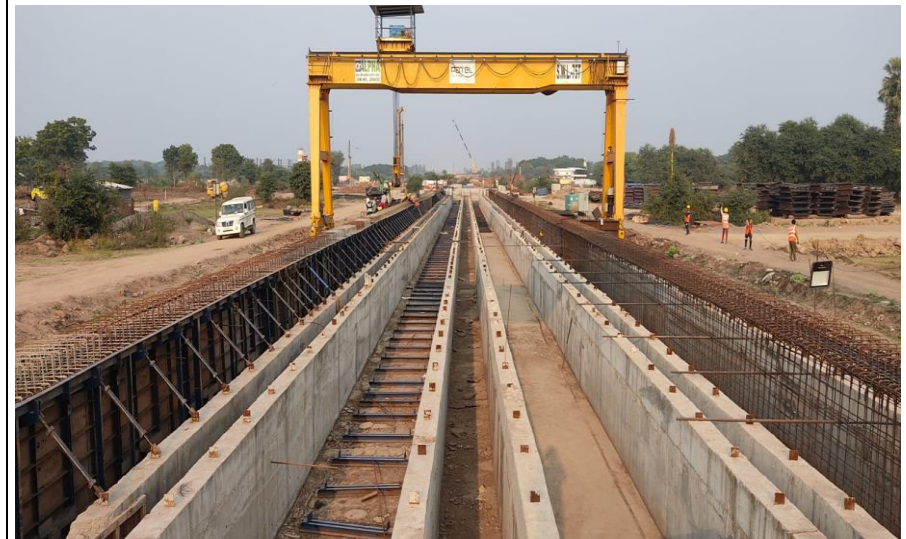
Shuttering & steel binding at Girder Casting yard
