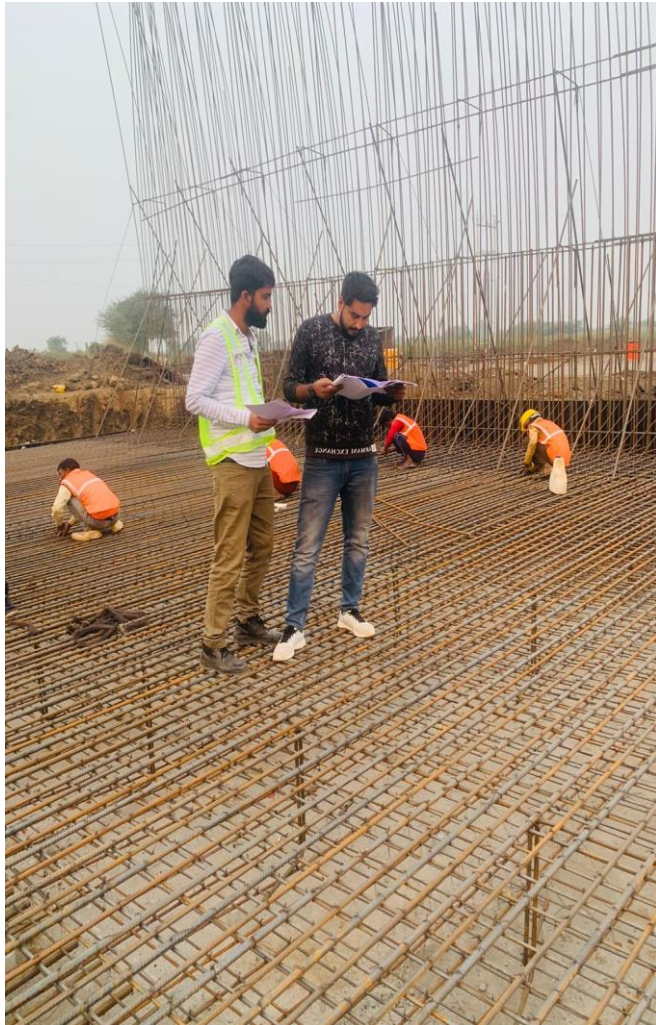
raft reinforcement checking by AE representative at LVUP
