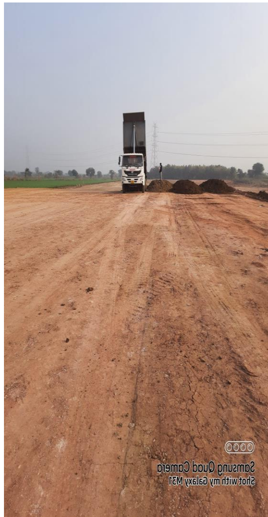
Embankment Dumping, Grading & Rolling
