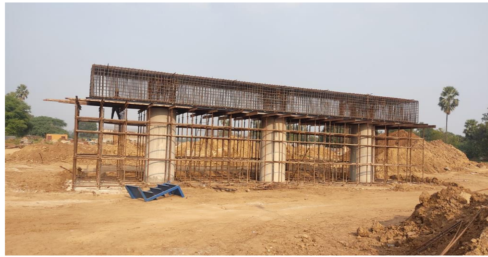
Reinforcement binding of Pier Cap MJB 352+281 Work in Progress
