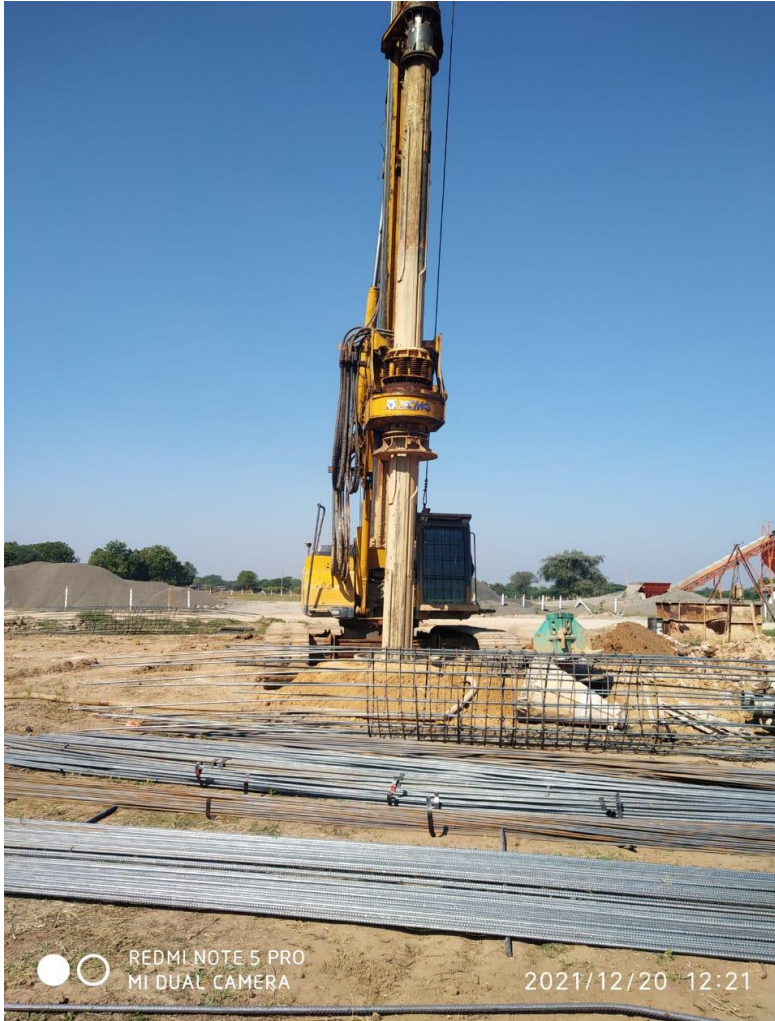
Pile Boring P34 pile No-1 at MJB 352+281
