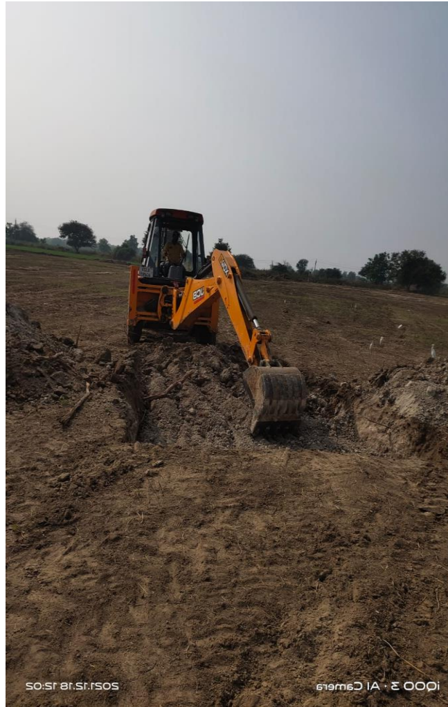
Excavation for BC at Ch-362+480
