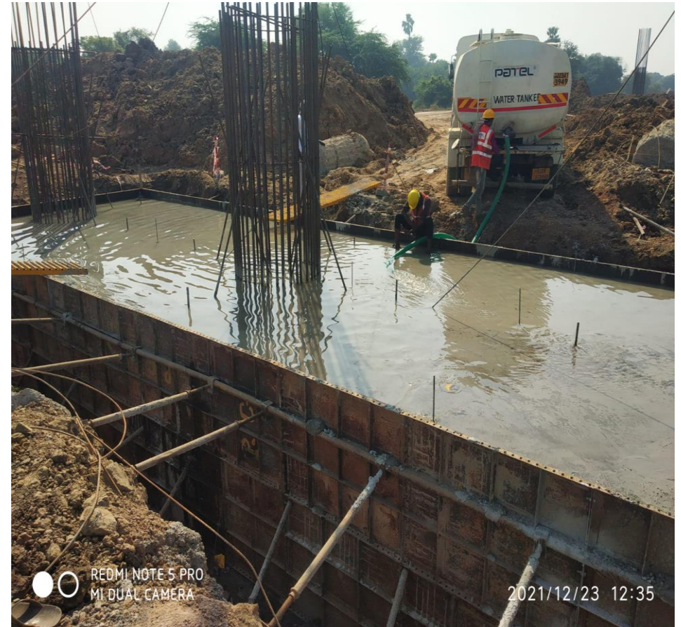
Pile cap P-34 LHS curing in progress at MJB 352+281
