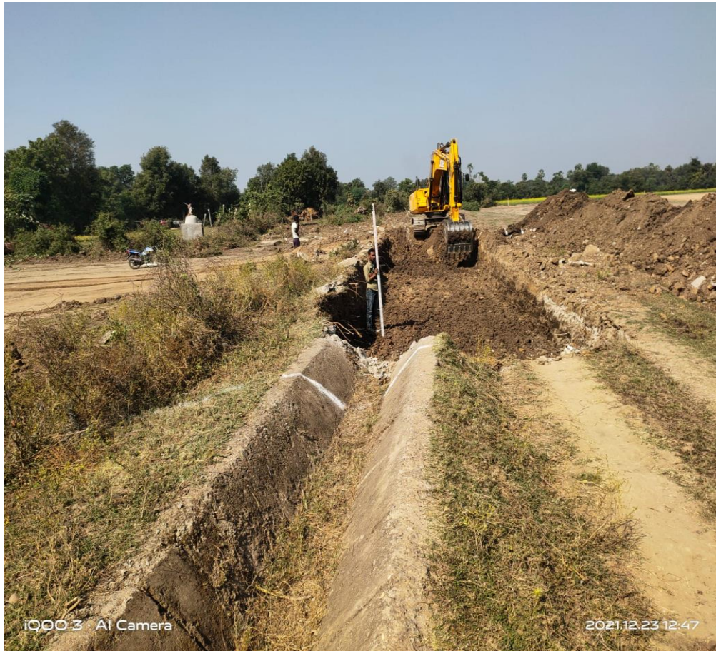
Box culvert excavation at ch.-356+465
