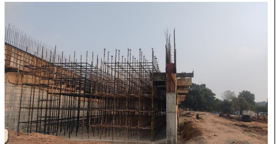
Staging & Shuttering WIP at LVUP
